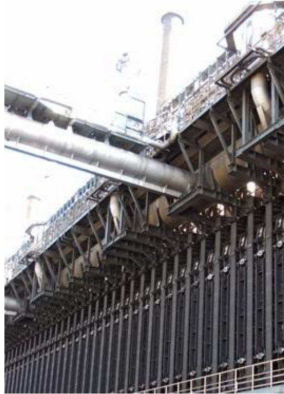
New coke oven battery 1E, Sumitomo Metals, Japan
