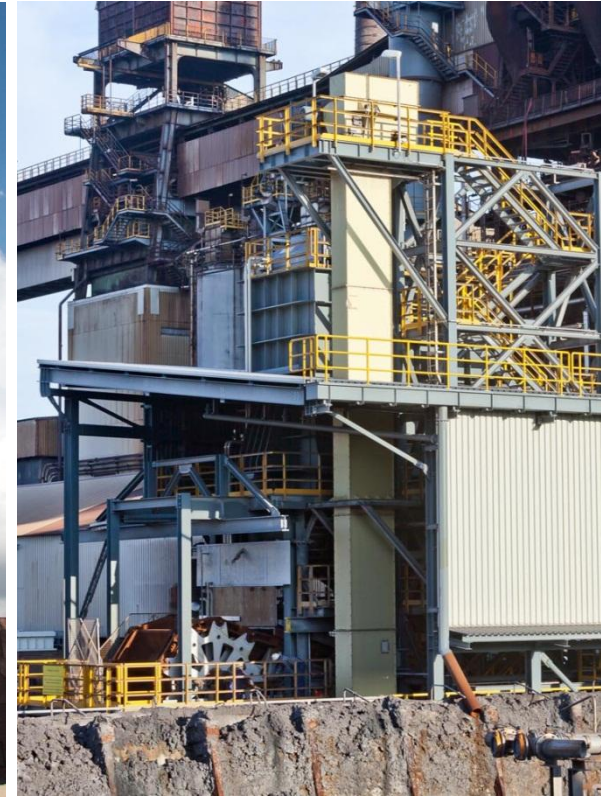
Dry Slag Granulation pilot plant, Dillinger Hütte, Germany
