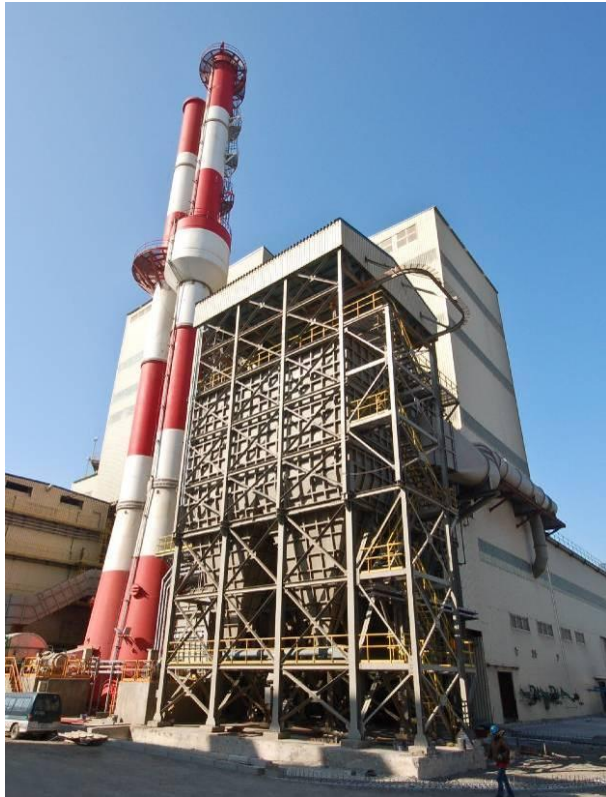
PRIMUS® recycling plant, Dragon Steel Corp., Taiwan
