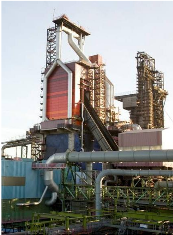
New BF8 with sub-plants, ThyssenKrupp Steel, Hamborn Germany
