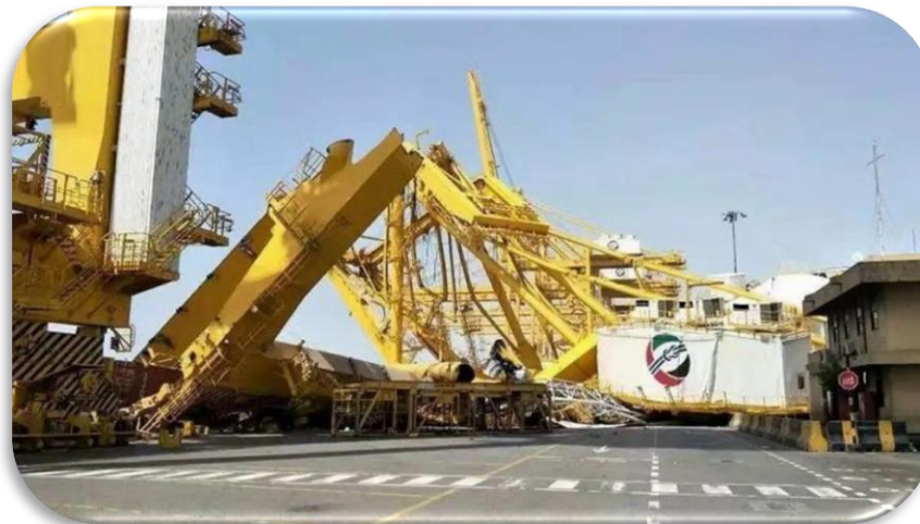
Crane collapse at Jebel Ali Port, Dubai
