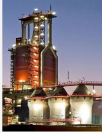
Blast Furnace Plants & Technology
